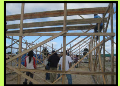
Putting up the frame.
